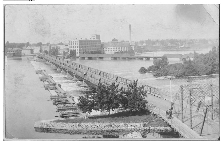
1893 – the 4<sup>th</sup> bridge was completed with an iron frame, wooden deck and a draw bridge allowing boats to pass; the cost was approximately \$40,000
