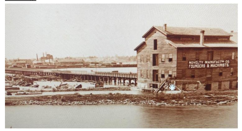
1883 – the 3<sup>rd</sup> bridge was completed; the bridge was about 7 feet above the water with a wood frame & decking; total cost was approximately \$10,000 paid for by the Town of Lawrence (west side of river) and De Pere (east side of river)
